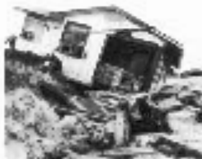
Figure 2.2. Flooding Caused This Foundation to Collapse
