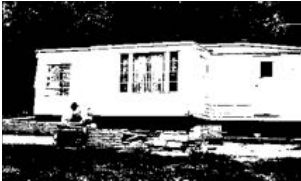
Figure 5-6. Failure due to sliding.
