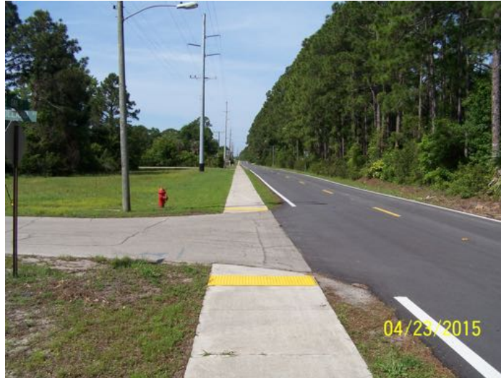
The sidewalk along Oak Street in Lanark looking west at the intersection of Holland Avenue.
