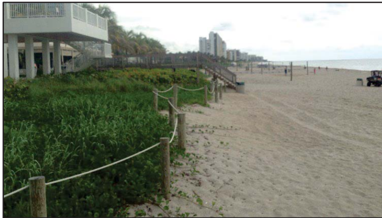
Figure 1: Post and rope fence constructed to state of Florida CCCL specifications. This pedestrian barrier rerouted foot traffic that was trampling newly installed beach dune plants and creating footpaths through the dune. Post and rope barriers are not to be run out onto the sandy beach and block lateral beach access.
